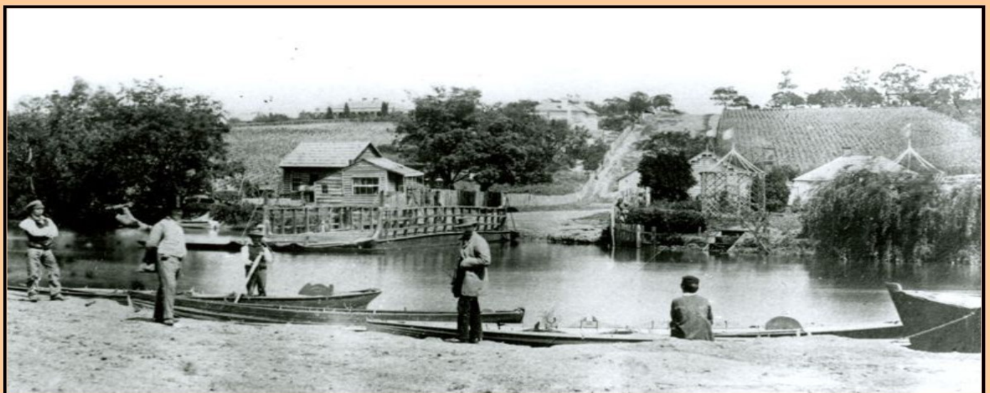
1856—WHERE PUNT ROAD MEETS THE YARRA RIVER
